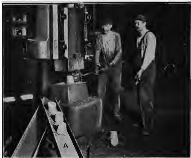
FIG. 4. UPSETTING THE BLANKS
